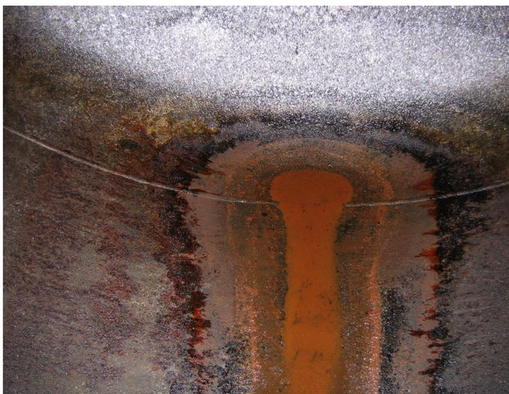
**Figure 4.** Example of corrosion that occurred in a rail car heel with poorly inhibited UAN.
